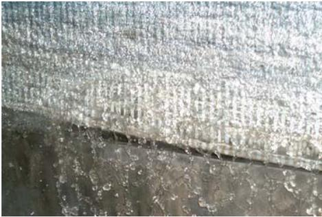
Figure 7. Water intrusion on the rolling face.
